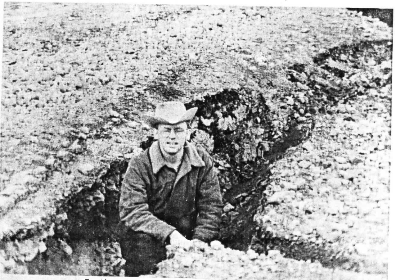
Earthquake damage near west end of runway "A"
