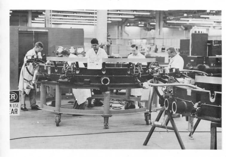
Once assembly is completed, the auxiliary launching ring is given a pneumatic test at 3,000 psi.
