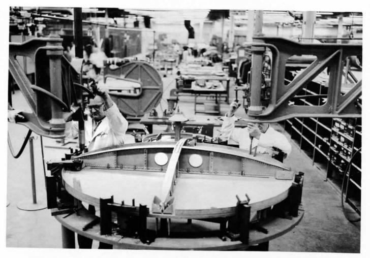
Another team builds up a pressure bulkhead, which is to be installed in the center of the aft section (neg. 31583).
