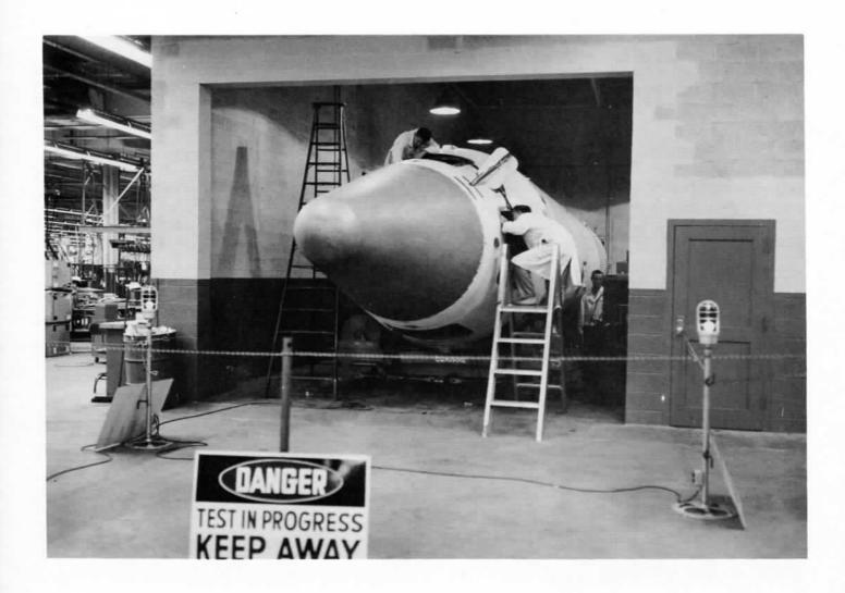
Pneumatic systems of JUPITER are checked out in this facility in a solidly-built, completely-equipped, enclosed area (neg. 31523).
