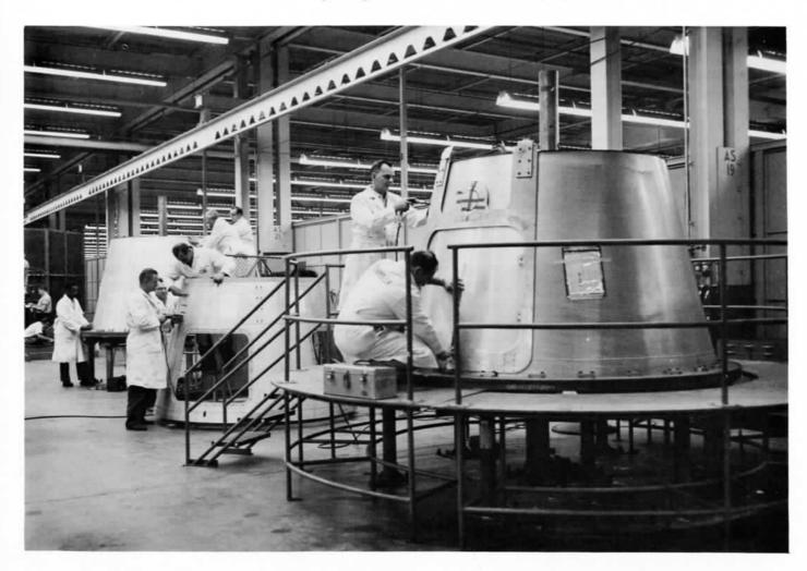
Workmen on assembly stands then apply their skill to completing details on this section by routing out four large holes. (neg. 31505).
