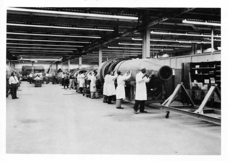
Nose cone and aft section for the REDSTONE consist of 8 longitudinal strips welded together around their frames. Men here finish up assembly of the skin section for the complete tactical body, or aft section of the missile (neg. 31533).
