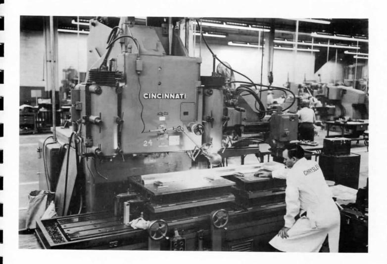
Another excellent machine tool is the Hydro-Tel, a profile mill which accurately follows a template (neg. 31584).
