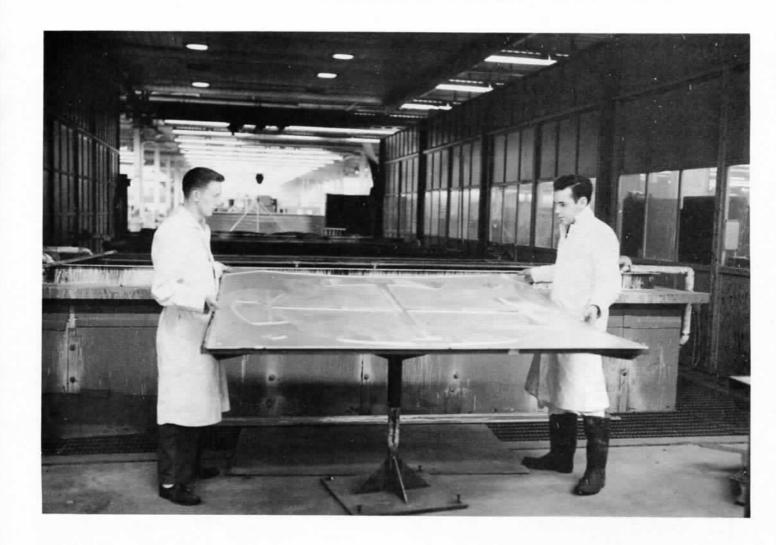
Another tank-type treatment available is chemical milling. With this equipment, selective etching of aluminum is achieved, as shown by this sample part (neg. 31552).
