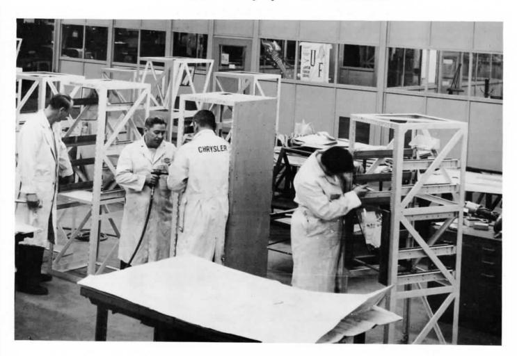
This is the final assembly area for JUPITER mobile and RIM area launching console racks. Electrical components are installed in the racks after they have been fitted into equipment trailers.
