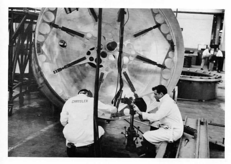
A supporting structure and other components are welded into the bulkhead (neg. 31556).
