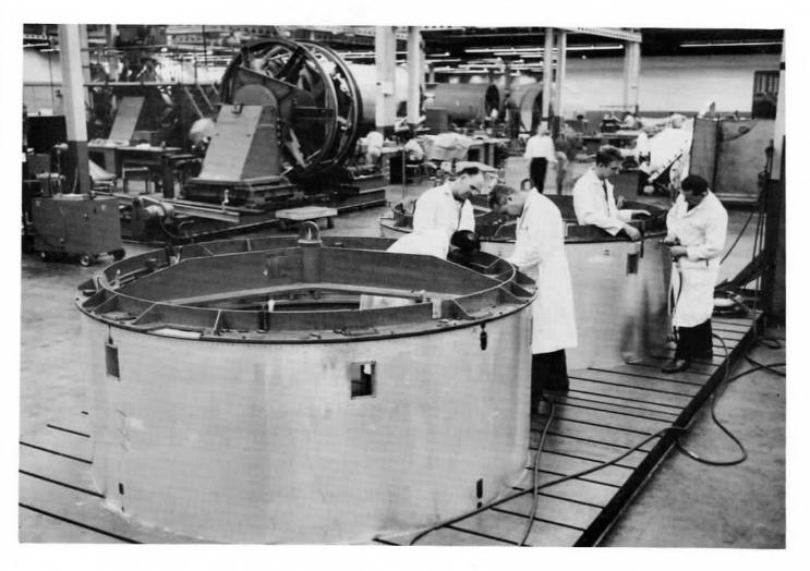
On the larger skins, assembly crews install vertical support brackets as well as Z-rings (neg. 31504).
