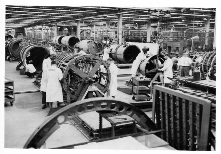
In another assembly area, the REDSTONE missile is also put together as three separate sections. Here, on the left, technicians make up the skin frame for the aft section, while at the right men are fashioning the nose cone (neg. 31532).
