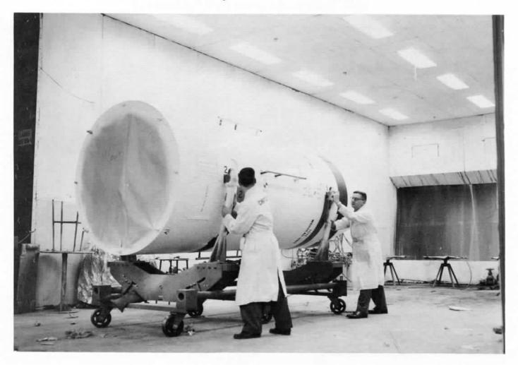
The tactical body, now completed, is rolled from the paint booth after receiving its new coat (neg. 31546).
