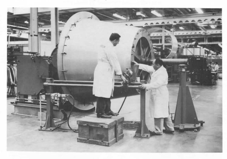
JUPITER IS BUILT UP AS THREE MAIN PARTS. On the aft or top section, the first step — after the half-round sheet metal pieces are welded into a cone — is to trim the "skins" section on this rotary fixture (neg. 31503).
