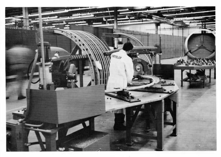
Support rings, or Z-segments for the skin sections, are trimmed to length with a power saw (neg. 31510).
