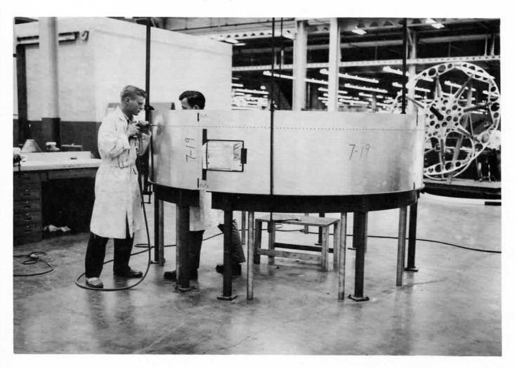
Two workmen rivet in a Z-ring on the shortest of the seven skin sections (neg. 31515).
