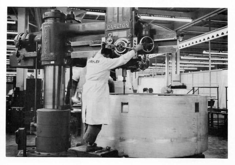
A big radial drill is brought into use to provide holes for joining Skin 1 to the aft section (neg. 31557).
